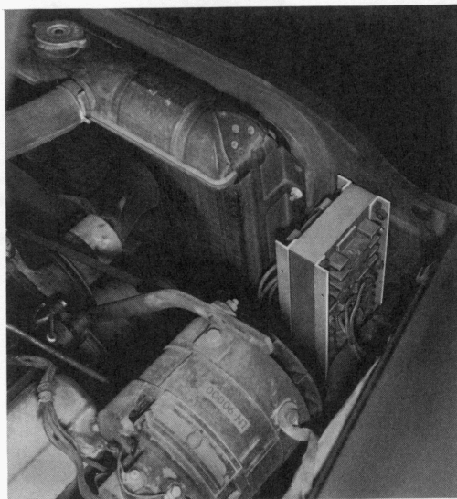
ENGINE COMPARTMENT VIEW of W8DLD's station wagon, showing Leece-Nevele alternator in foreground and 3-phase distribution transformer mounted just ahead of it next to radiator.
