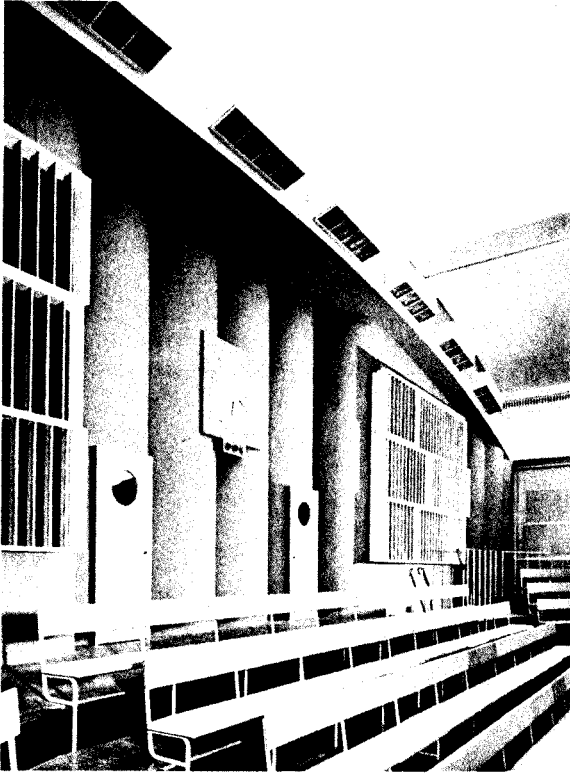
FIG. C/18. Maida Vale Studio 1. Back wall showing dispersive treatment and organ grilles. Part of the permanent choir seating is also shown.
